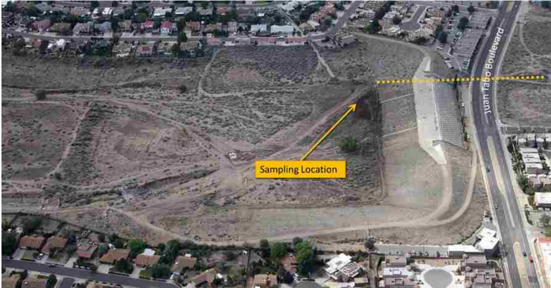
Figure 7: Sampling location in the fore bay of the John B. Robert Dam, Aerial Photo Courtesy of Eagle Eye Photography
